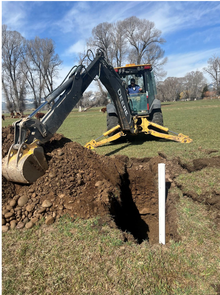
Photo 2: Groundwater monitoring piezometer installation JG-2
