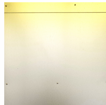
4. MATTE FINISH SILVER SHEET METAL 22 GAUGE FLAT EXPOSED FASTENERS
